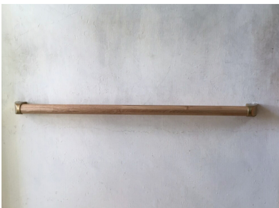
Installation of handrails in the living room
