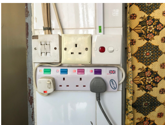
Replacement of malfunctioning extension cord
