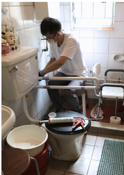
Installation of handrail
